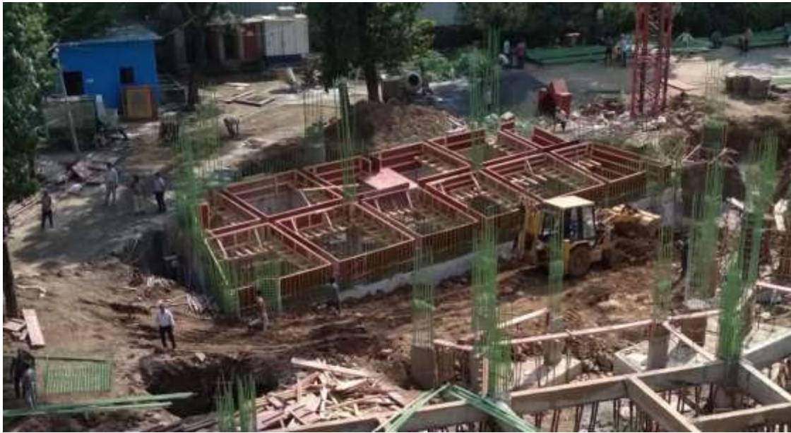
Rain Water Harvesting facility under construction in 2022-23
