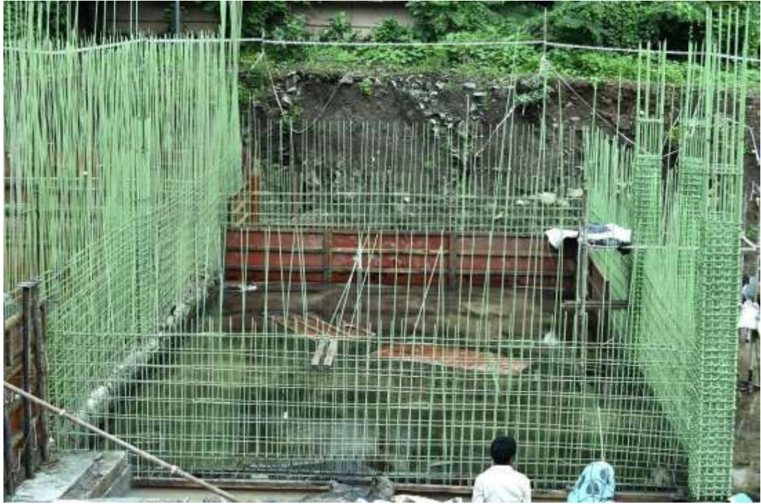
Rain Water Harvesting facility under construction in 2022-23
