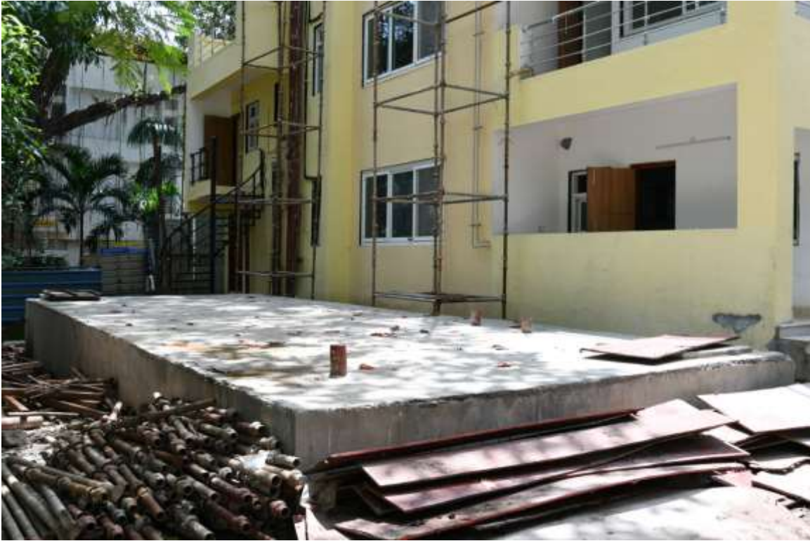
Underground Water Tank
