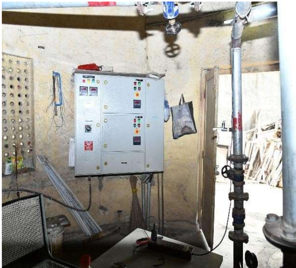
Bore Well Pump House
