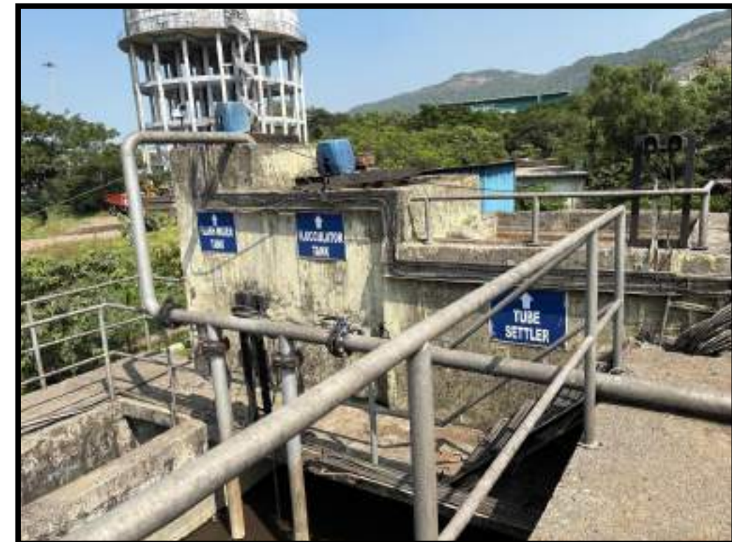
Fig. 6 Tube Settler
